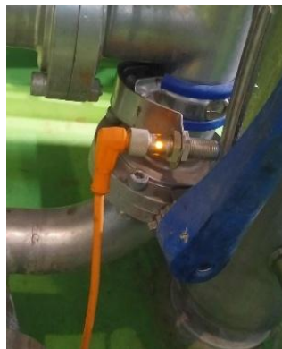
Gambar F.2 posisi pemasangan sensor proximity inductive
