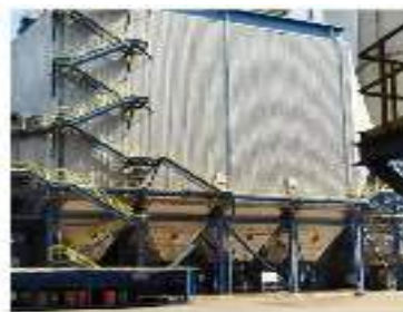
Gambar 2. Electrostatic Precipitator System PLTU
