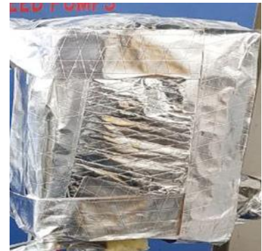
(Figure 4) shows the water tank.
