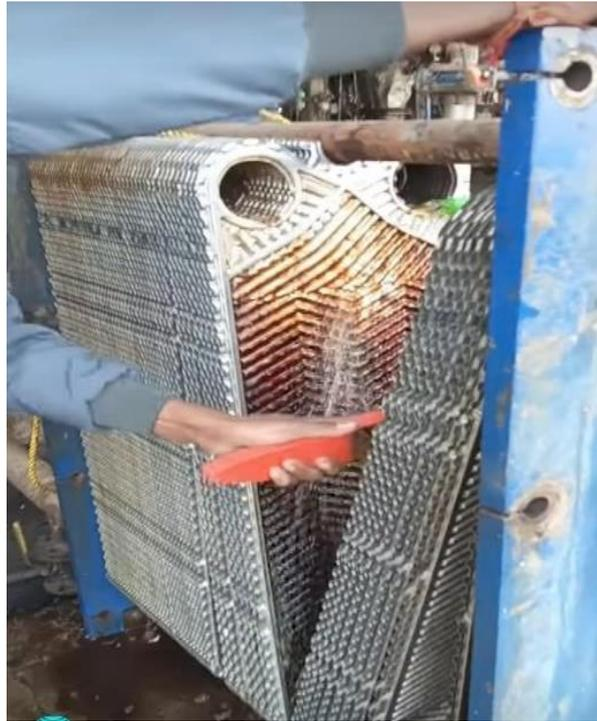
**Gambar 4.** Proses *Mechanical Cleaning* PHE
