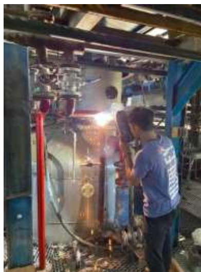
Gambar 1. Proses perbaikan pipa steam
