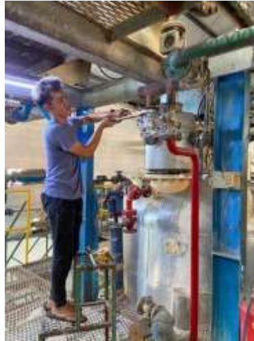
Gambar 2. Proses penggantian kran pipa steam
