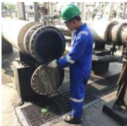
**Gambar 5.** Pengecekan dan Pembersihan *Shell* Heat Exchanger E301
