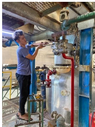
Gambar 2. Proses penggantian kran pipa steam
