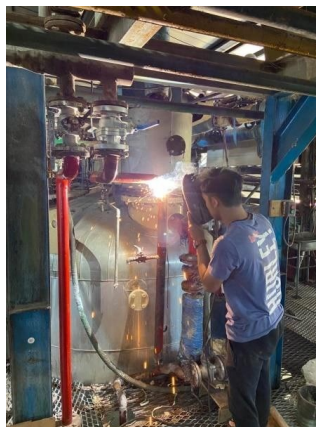
Gambar 1. Proses perbaikan pipa steam
